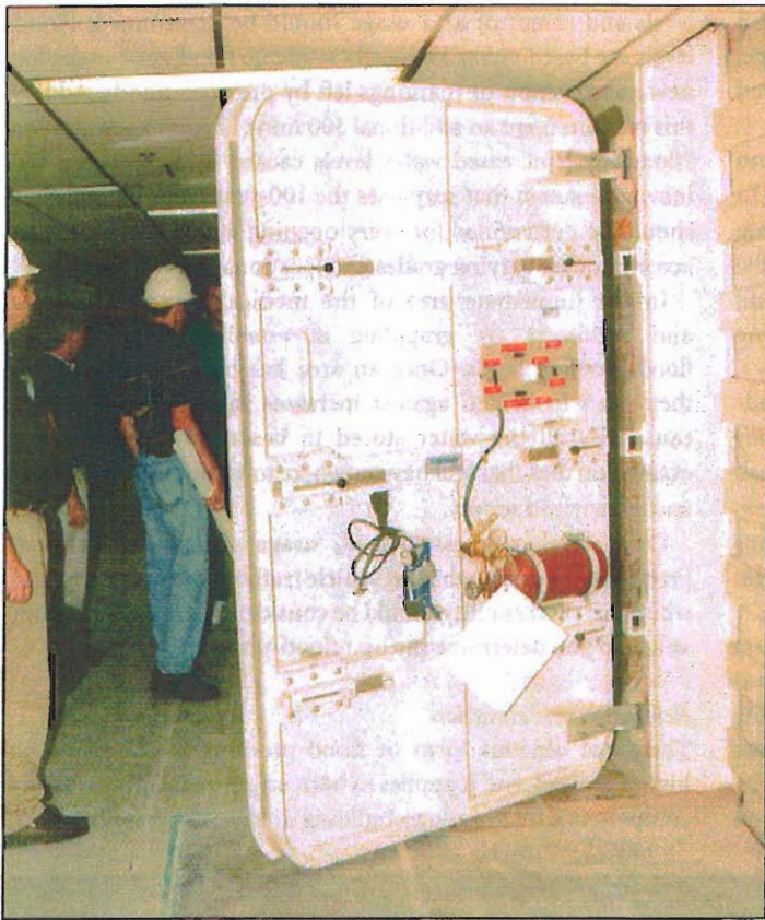
Bulkhead doors are watertight and protect entrances to basements, tunnels, and galleries, and can be designed to provide total protection under meters of standing water.
